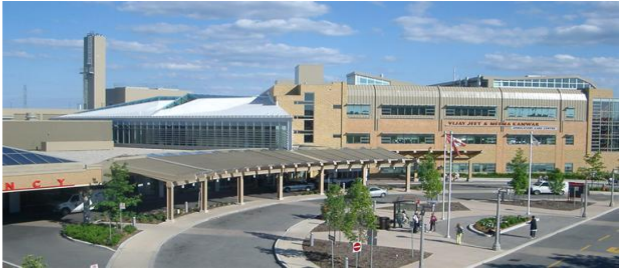
Picture 1. Credit Valley Hospital
